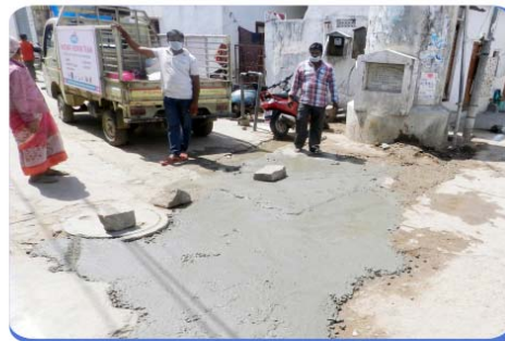
Repair Road at Masjid Circle Vemukunta (After)
